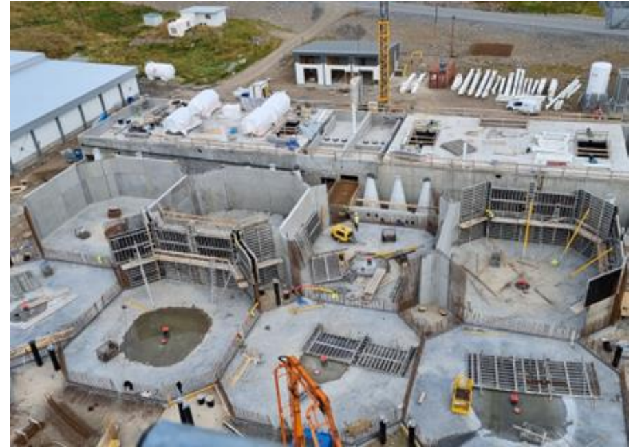
Current progress in Norður Botn
